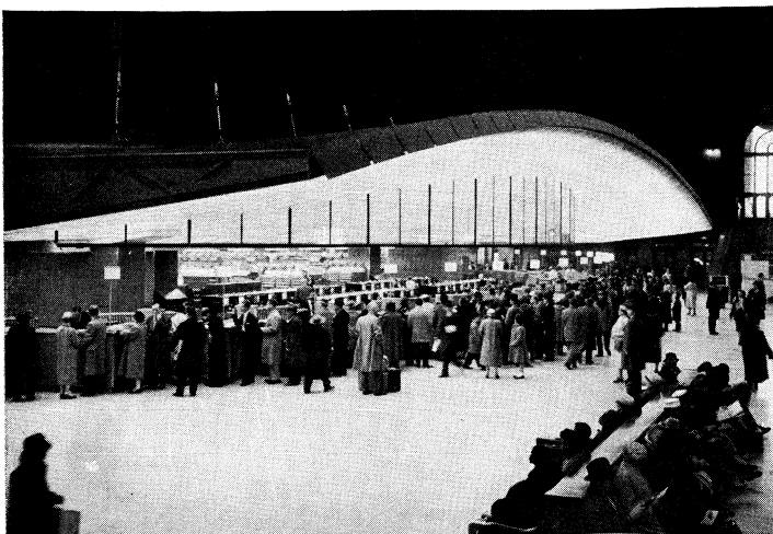
Remodeled ticket counter in the Pennsylvania station, New York city. Electronic devices, including television, were added to facilitate reservation handling
