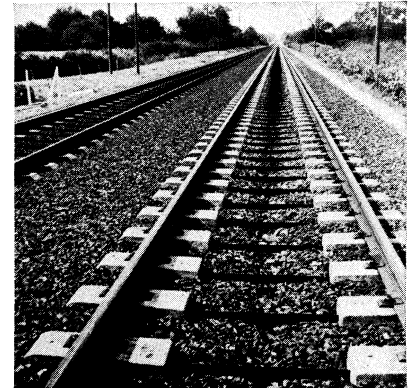
A modern roadbed: long welded rails set into concrete and steel cross-ties (sleepers)
