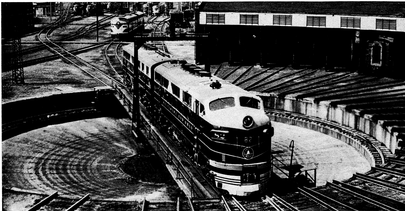
Turntable and roundhouse where locomotives receive cleaning and light repairs. Dieselization of American railways eliminated many such roundhouses originally built to provide the frequent maintenance required by steam locomotives
