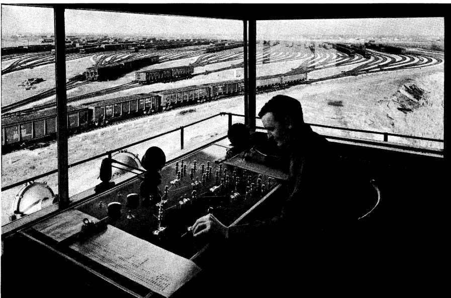
Control tower in the Markham, Ill., yard of the Illinois Central railroad. As freight cars roll down a hill, operator punches buttons to direct each car or group of cars to its appropriate classification track. Electronically controlled retarders regulate speed of the roiling cars
